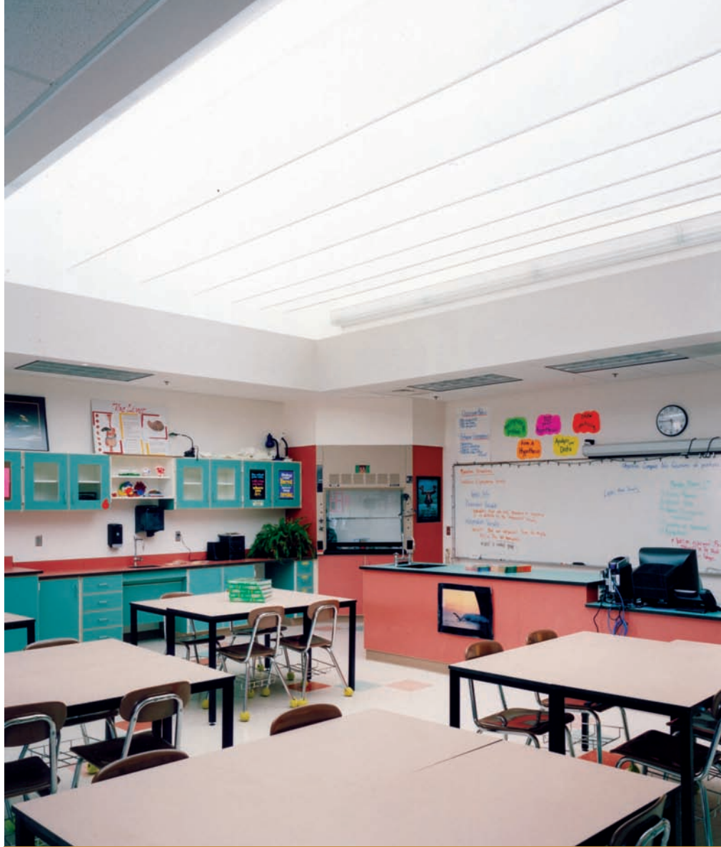
Baffles inside south-facing monitor.
