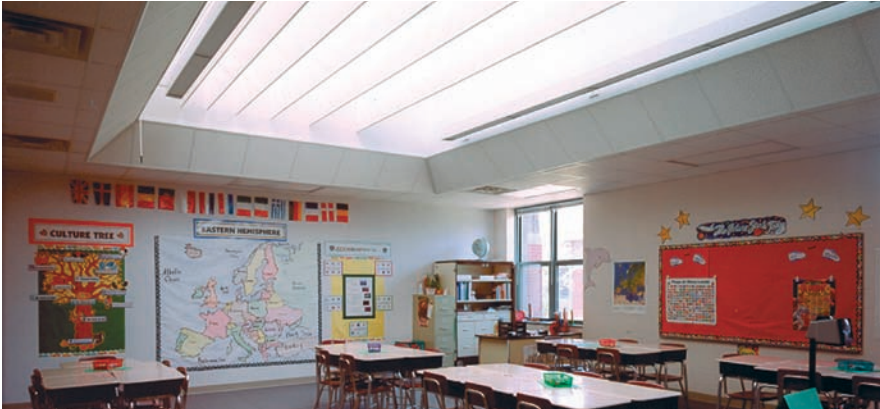
Durant Road Middle School was constructed under budget. The first year savings attributed to the daylighting and roof assembly were over $0.50/ft 2 . The additional cost for the 150,000 ft 2 facility was $115,000, and the simple payback was less than two years.
