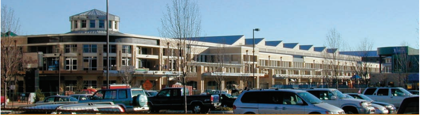
For Chattanooga Convention Center, south-facing roof monitors provide natural lighting into the 100,000 ft 2 main exhibit area. The daylighting strategy and color selection reduced the load by 40 tons in just this one space.
