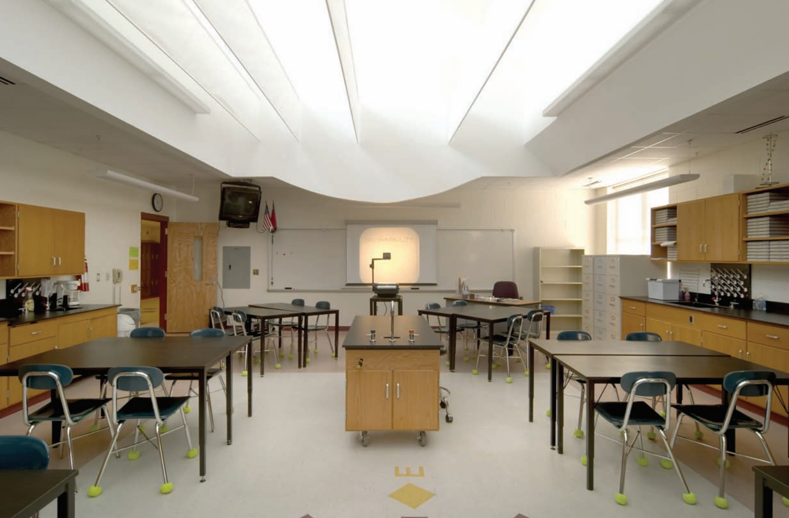
Architectural detail intentionally darkens the projection screen while still allowing daylight to the rest of the classroom.
