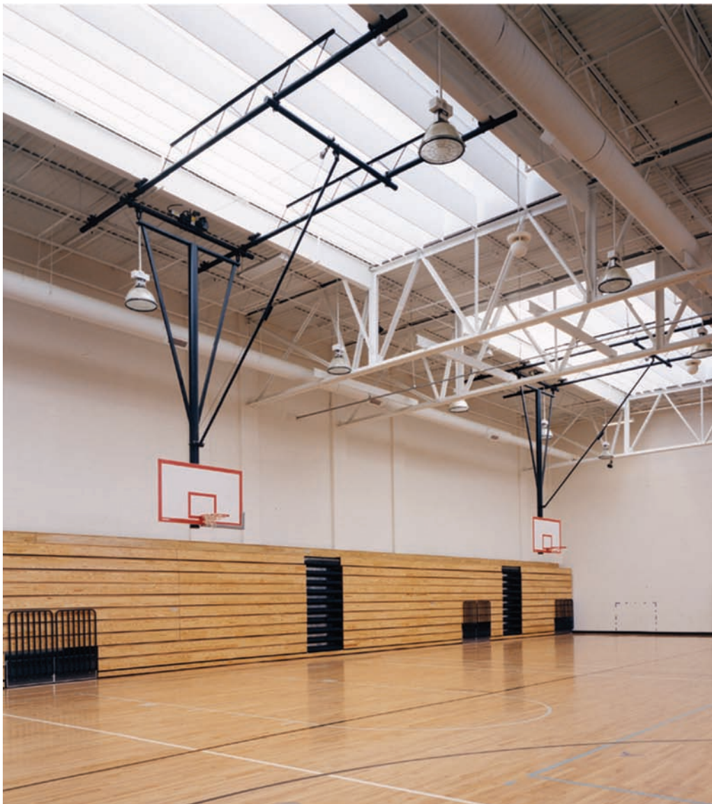
The south-facing monitors with baffles provide daylight to the gymnasium.
