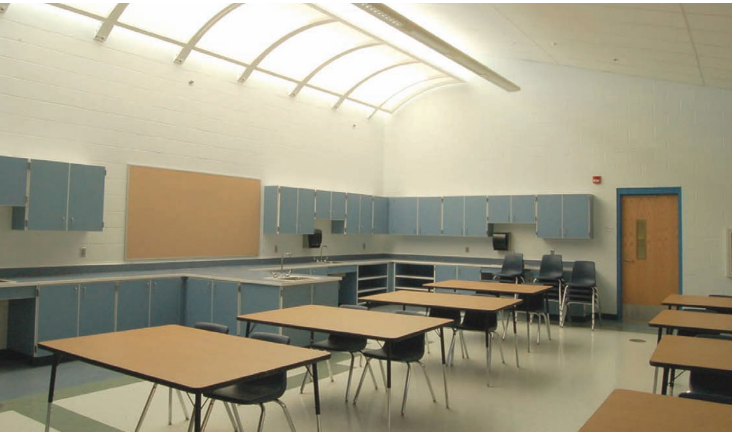
High ceilings and an underfloor air-distribution system allow hot air to stratify and condition lower spaces in the room.
